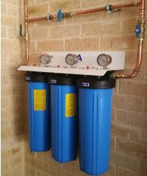
The Outdoor Systems are UV resistant however where possible it is best for the longevity of the system to install the unit undercover, or construct a simple cover for the system to shield it from direct sunlight and weather extremes such as rain, storms and frost.
