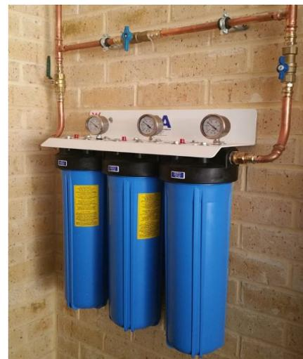
The Big Blue Systems are UV resistant however where possible it is best for the longevity of the system to install the unit undercover, or construct a simple cover for the system to shield it from direct sunlight and weather extremes such as rain, storms and frost.
